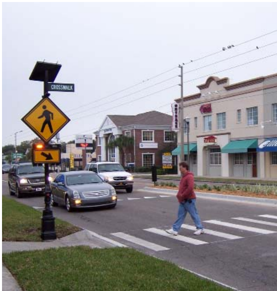
Rectangular Rapid Flashing Beacon (source: www.pedbikeimages.org/mf )
