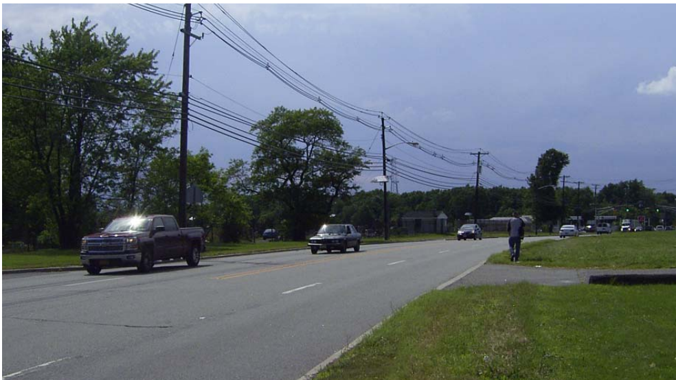
Lack of Sidewalks on Pfeiffer Boulevard
