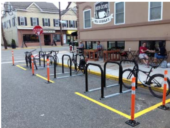
Flexible Bollards with Parking
