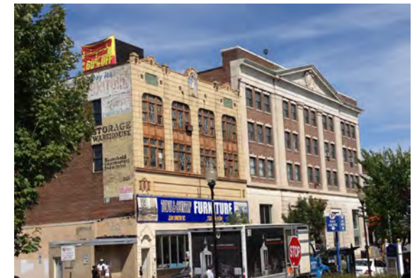
Underutilized upper floors along Smith Street
